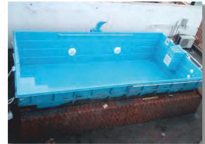
4. Make Brick wall around the Swimming pool.
