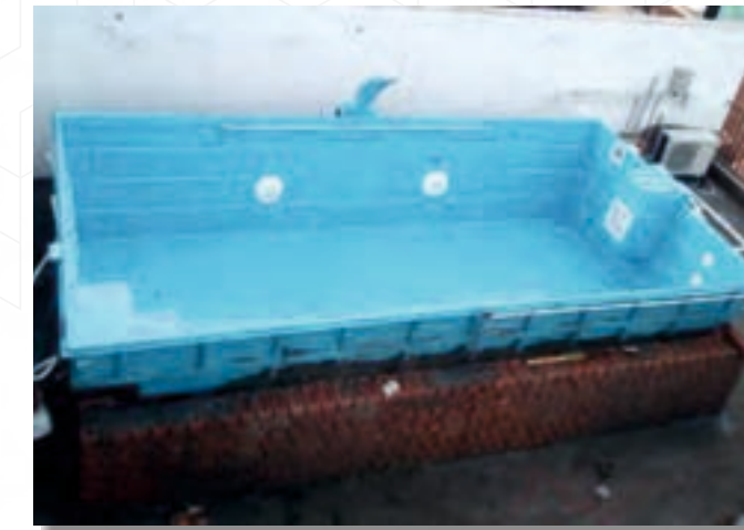
4. Make Brick wall around the Swimming pool.
