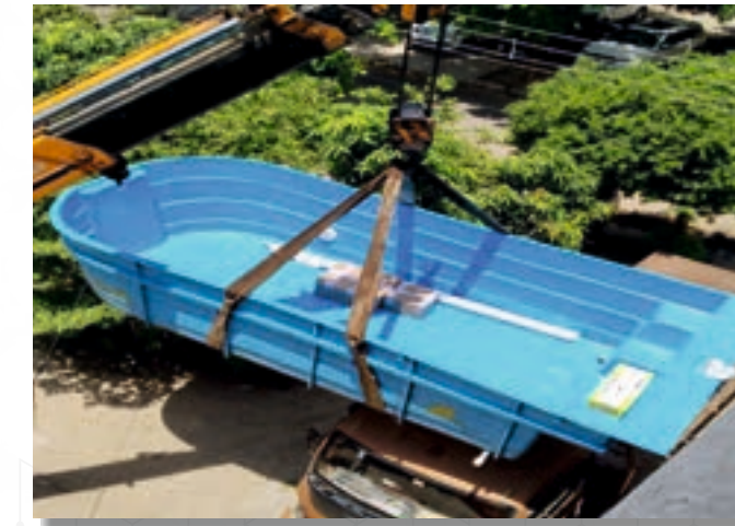
2. Placing the pool with the help of Crane at site.
