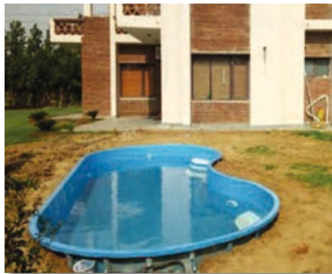
5. Filling water in pool and make deck area.
