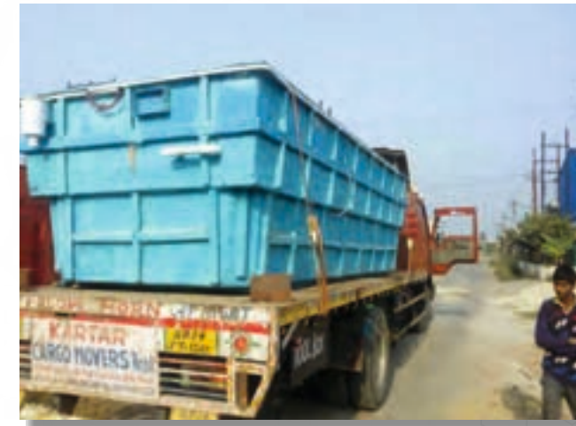
1. Transportation of Swimming Pool via Truck.
